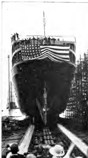
The Southern Pacific Company's steamer Bienville sliding off the ways at the yard of the Todd Drydock & Construction Corp., Tacoma.
